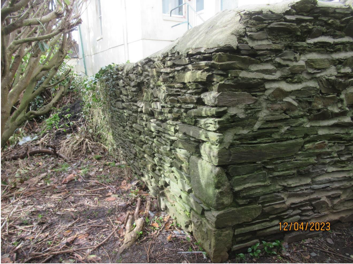
P7 – west boundary wall
