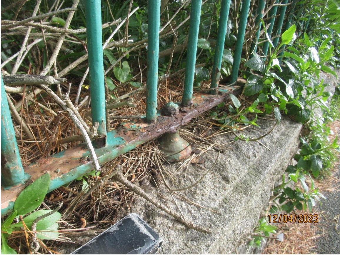
P16 – base of railings
