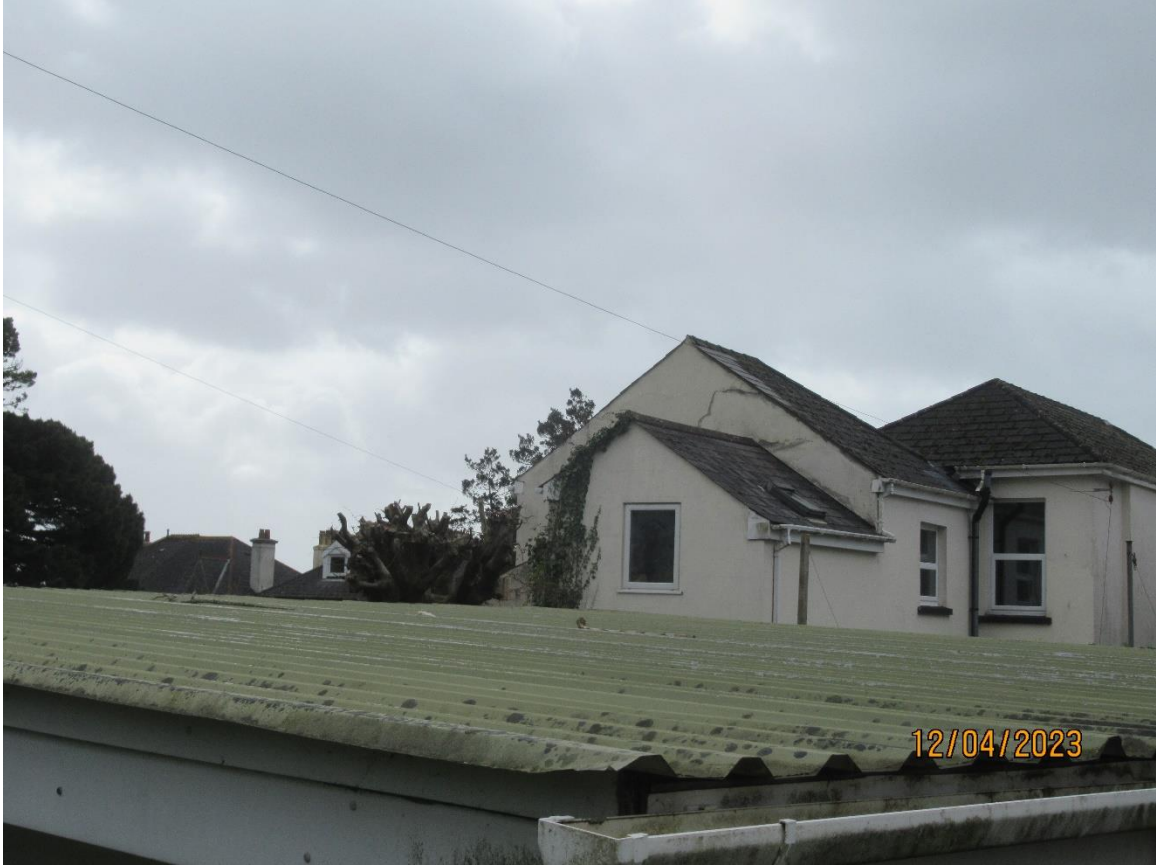
P23 – roof to Maurice Huggins room
