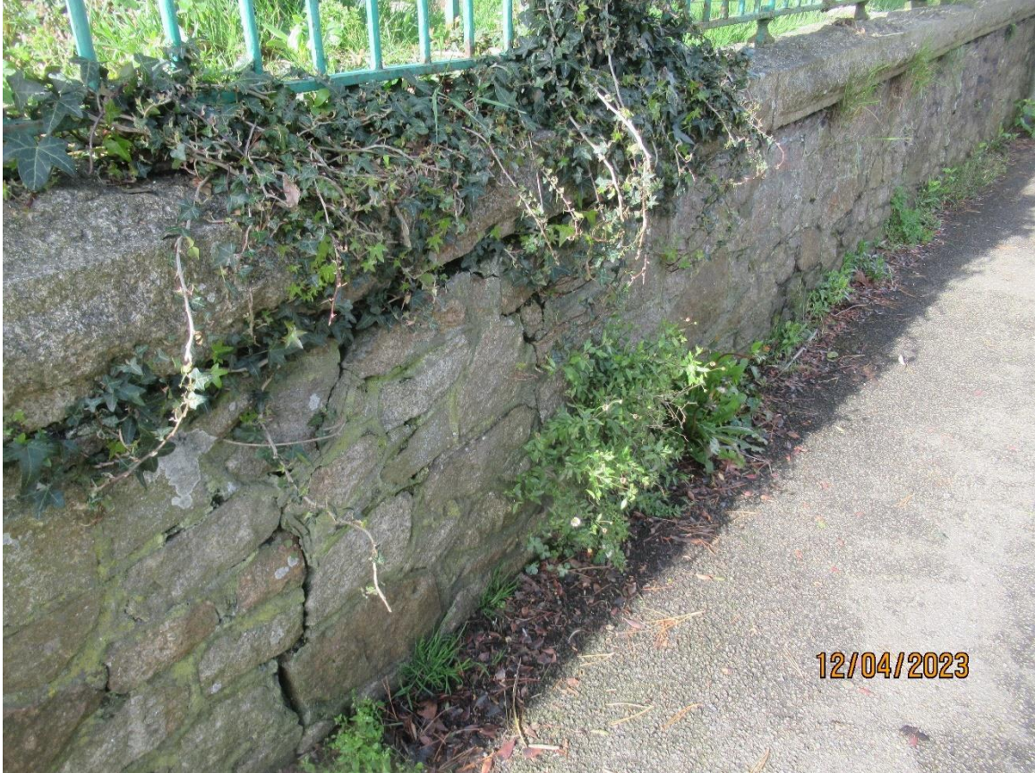
P4 – rotational displacement near tree
