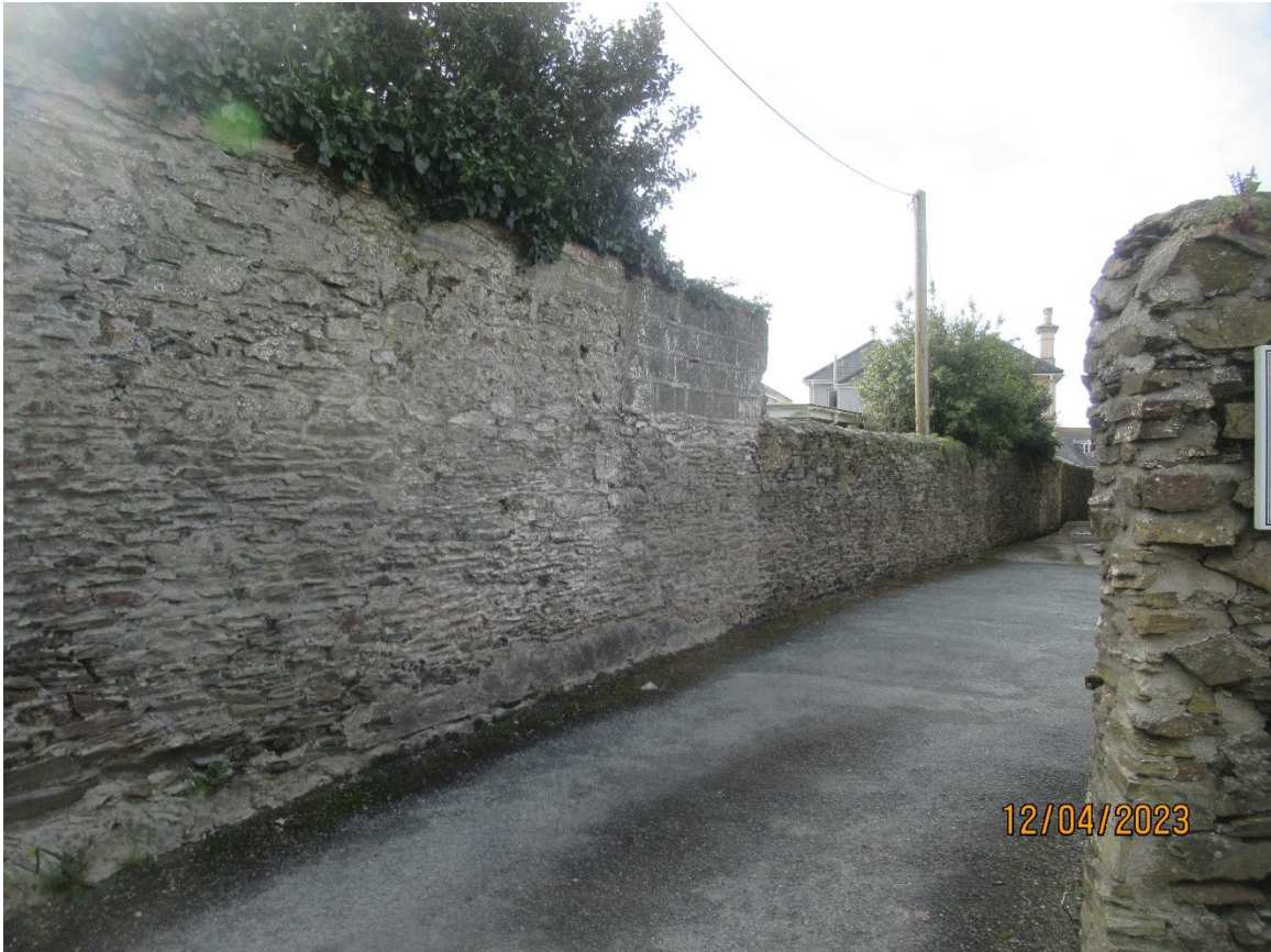
P9 – west boundary wall
