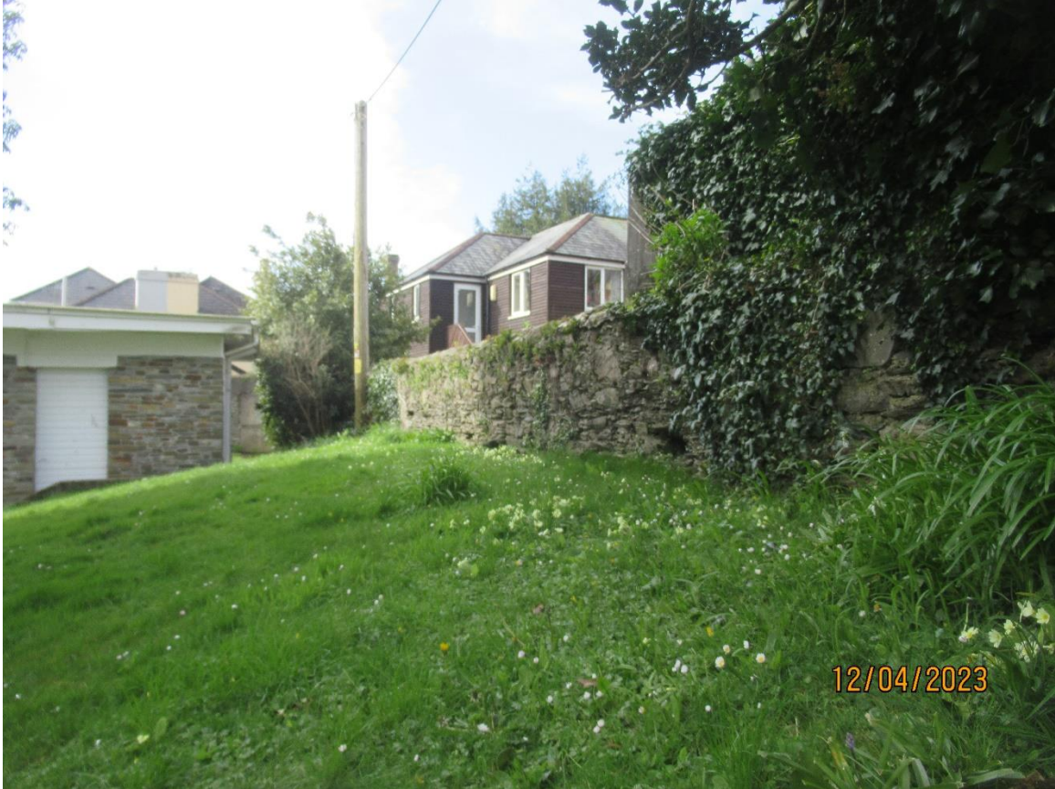
P8 – west boundary wall
